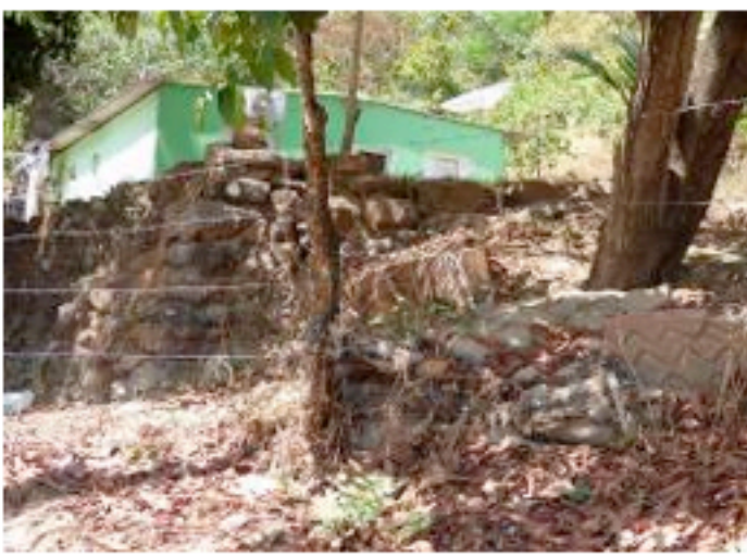
Figure 2 – Riprap ground on the slope of azul saw Source: Author's photo (2015)
