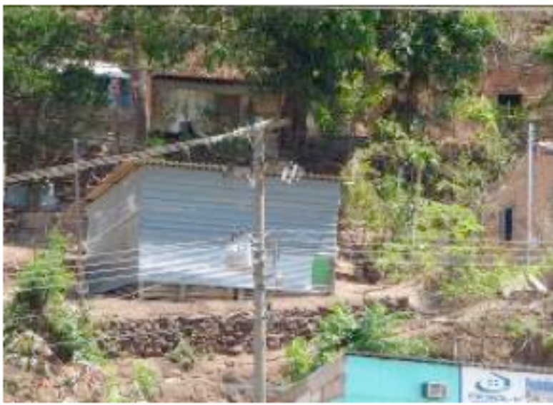
Figure 11 – Building with improvised materials. Source: Author's Photos (2015).
